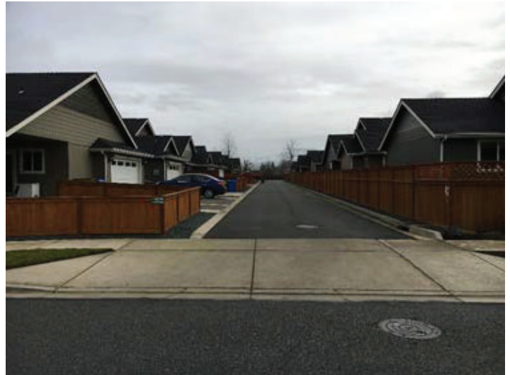
New alley way enhances neighborhood connectivity paralleling Elmer Nelson Lane
