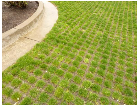
Figure 4-52. Concrete grass pavers are great for overflow parking areas to preserve site permeability in low traffic areas. (In high traffic areas, grass and turf will be shaded too much to grow grass. Use gravel in this case.)
