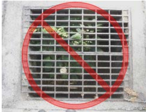
Figure 1-21. This catch basin has so much sediment a shrub is growing in it.
