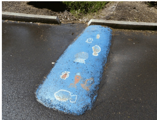
Figure 4-67. For curb cuts on a slope, one effective means of turning the water 90-degrees into the facility is to pour an extruded speed bump-type structure onto existing pavement just downstream of the curb cut. Decorating this structure with fish is not necessary, but certainly raises awareness of the facility behind it.
