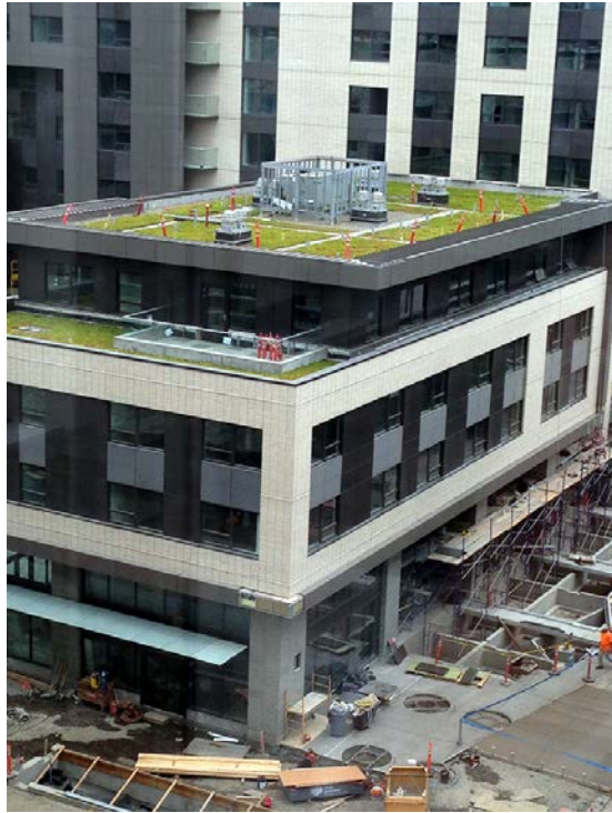
Figure 4-34. Carefully protect the vegetated roof at all times through the construction process through signage or other means. A variety of contractors, not directly related to the vegetated roof installation, could damage it.
