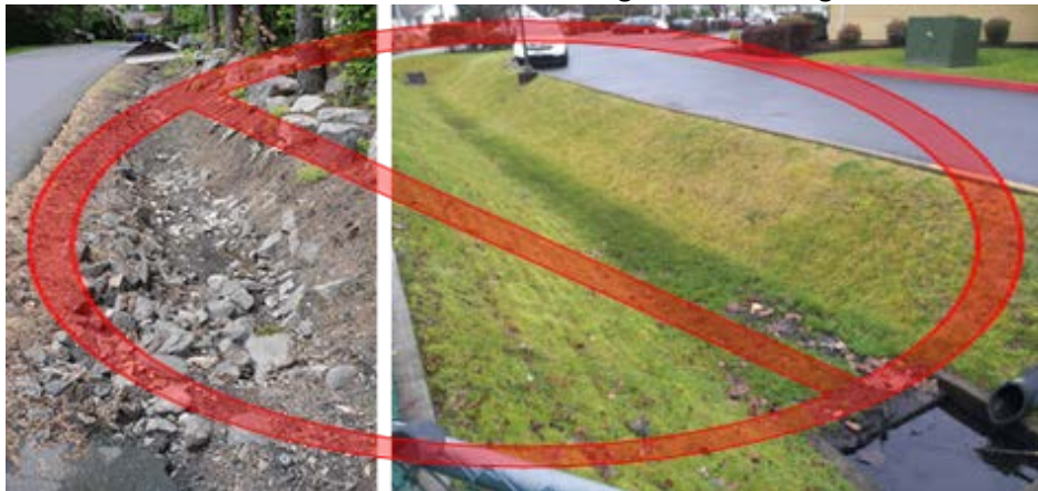
Figure 4-95. Roadside ditches (left) and grassy mowed swales (right) are common ways to convey stormwater; however, without tall, densely planted vegetation and a design to protect against erosion, these swales are more likely to pollute water, not treat it. These facilities are even more undesirable when relied upon as an “end-of-pipe” solution, located at the bottom of the site, which is generally not considered LID because BMPs should be distributed around the site. Ideally the high side of a site will have as many BMPs as the low elevations.
