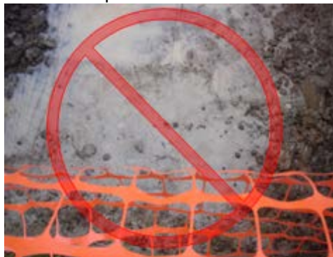
Figure B-11. Fine clay particles exposed to rain fall have re-sorted and clogged this infiltration facility.
