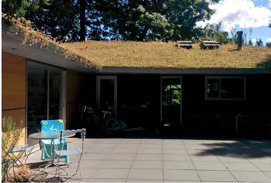
Figure 4-33. Irrigation was not installed on this vegetated roof and no supplemental water has been applied to the roof in a number of years since its establishment. This is acceptable for the chosen plant palette. The vegetated roof will regain its green color when the rain returns. This roof has considerable shade from existing tall trees much of the day.
