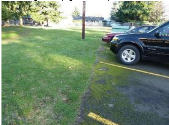
Figure 4-106. The parking lot sheds runoff to the left towards the grassy area. A lack of curb and flat area means almost all the annual runoff from the parking lot stays on-site.
