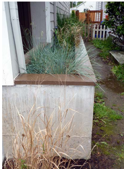
Figure 4-57. A residential above-ground stormwater planter. This facility is lined to prevent infiltration too close to the basement.
