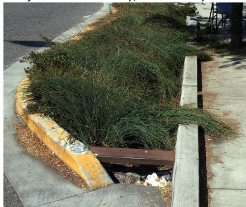
Figure 4-68. A "bumpout" style rain garden where the curb drains directly into the facility without having to change the direction of its flow is a good application for a curb cut. A metal bar across the opening provides a mild warning, approximately equivalent to a curb, to alert drivers who might pull forward into the facility.
