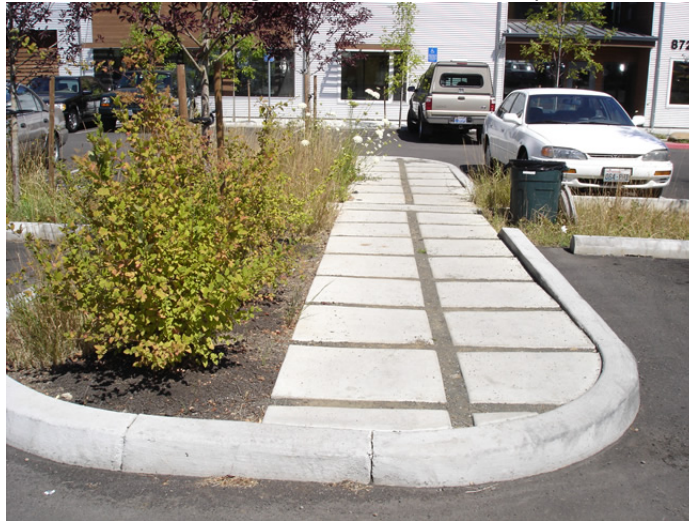
Figure 4-53. One cost-effective solution for permeable pavers is this poured-in-place installation. Two-by-four lumber was used to create a grid on top of the base rock and conventional impervious concrete was poured between them. After curing, the lumber was removed and the gaps were filled with infill rock. (See Detail BMP 5.04.)
