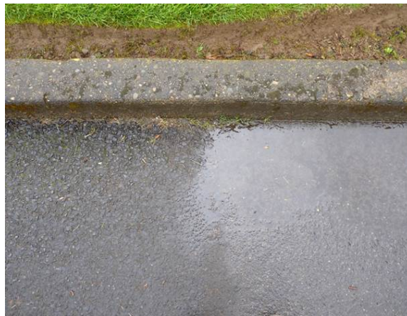
Figure 4-43. Porous asphalt (left) was installed next to impervious asphalt (right) in a public street to solve flooding in a very flat area.
