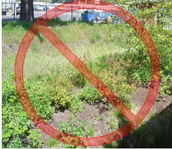
Figure 4-98. This WQ conveyance swale was squeezed into a constrained space by snaking it through available space and compacting the sides to create slopes that exceed 3H:1V. While many plants were successfully established, many steep slopes remain bare (foreground right and background left).
