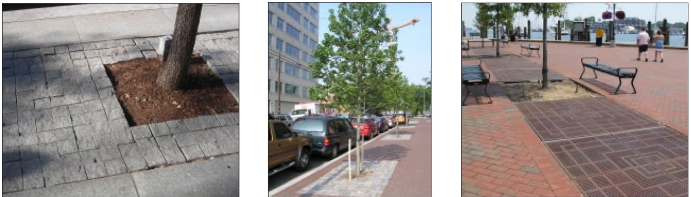
Figure 4-23. A variety of pavements, both impervious and permeable, can be used to create a covered tree space. Pavers, such as granite cobbles and permeable paver blocks (shown above left and middle), placed with gaps between the stones allow water to flow to the soil below. Grates can be used as a soil covering when they are not immediately adjacent to the tree. Photos courtesy of Casey Trees.
