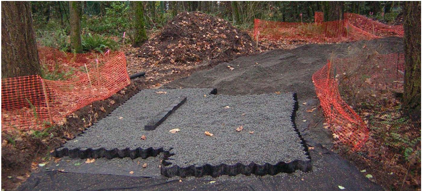
Figure 4-41. The grids of a flexible paving system can be seen on the edge here. In this case, the flexible paving system reduces the depth of excavation otherwise needed to install permeable pavers (which sat on top of this system at the end of construction). Reducing excavation, among other best practices such as careful root pruning (see Chapter 4 “Tree Protection BMP”), protected the health of the two trees pictured on either side of the roadway.
