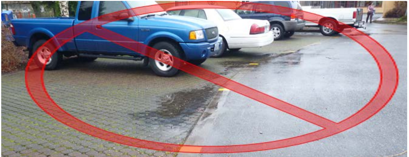
Figure 4-37. Impervious pavement is tipped toward the permeable pavers, which has clogged the entire first few feet of the pavers. Where the pavers were not installed flat, ponding makes this clogging evident.
