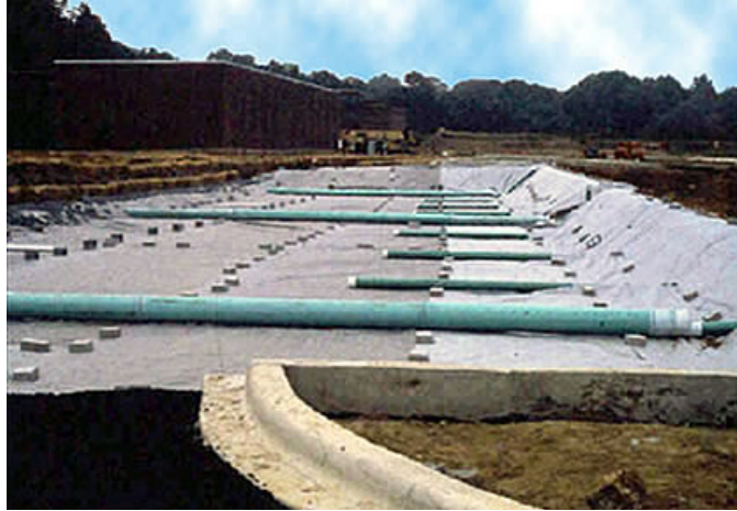
Figure 4-51. Non-perforated pipes convey runoff from uphill impervious areas to the perforated pipes pictured here at the bottom of the porous pavement before gravel has been placed.
