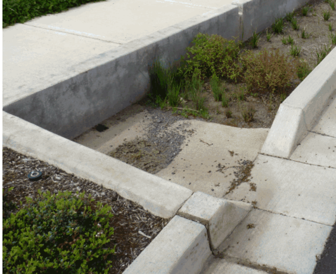
Figure 4-65. This concrete pad is tipped slightly away from the vegetated stormwater facility in the background and shaped with a slight off-center dip. As evidenced by the sediment, this pad works relatively well as a pretreatment strategy, but some dirt can be seen washing into the planted area, which is not ideal. This pretreatment strategy is suitable for medium sediment loads.
