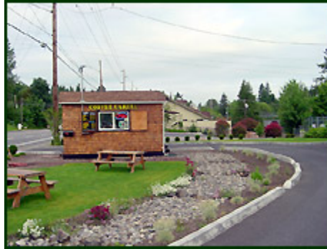
Figure 4-85. Soakage trenches receiving flows directly from the surface (photo courtesy of Lower Columbia River Estuary Partnership)
