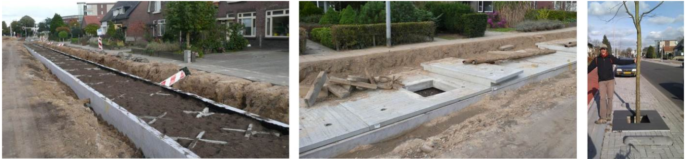
Figure 4-27. The same elevated pavement in a parking area during three different stages of development. (Left and center photos courtesy of Jim Labbe. Right photo courtesy of Jeff Mandel.)
