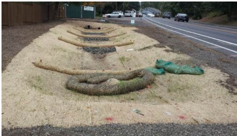
Figure 4-82. This image shows a great example of erosion prevention and sediment control for an LID swale in the public right-of-way after construction but before planting.
