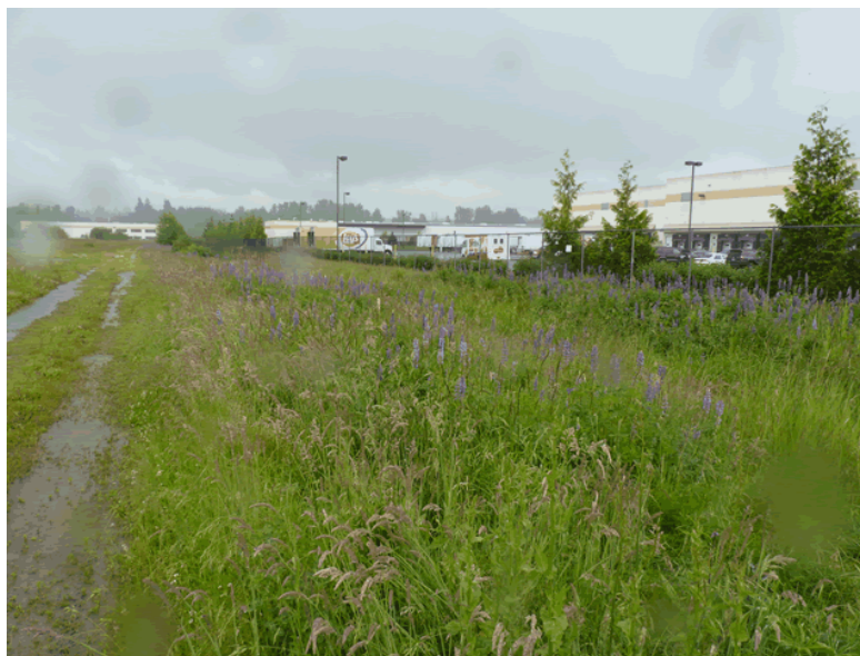
Figure 4-100. Vegetation is tall and sturdy enough to withstand flows during this rain event. A variety of plant species including lupines and grasses are included in this swale and add beauty. If mowing is required by ODOT, include a geogrid on the bottom to stabilize the surface for mowing.
