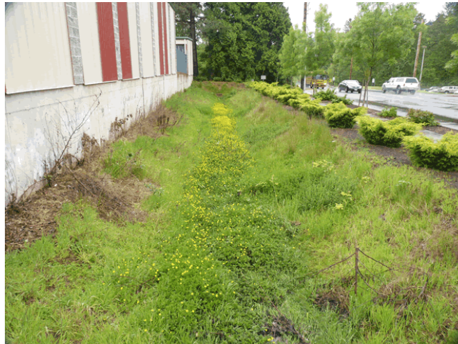
Figure 4-96. Partially or fully lined facilities may be located next to buildings; however, they will be more costly to construct (see “Cost Considerations” below).
