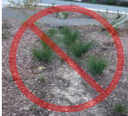
Figure B-8. This facility is being eroded and exporting sediment off-site. A high-flow bypass or better plant placement and establishment could help.
