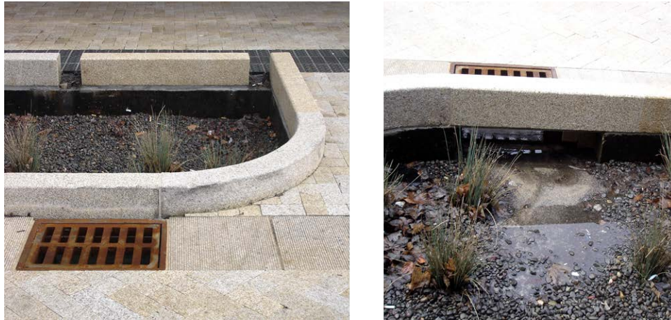
Figure 4-69. The front (left) and back (right) of this inlet is pictured. This is one way to avoid using curb cuts when flows along a curb need to be captured and redirected. Add a sump to the catch basin inlet to capture sediments, seen on the right, for a lower maintenance strategy for settings with medium and high sediment loads.
