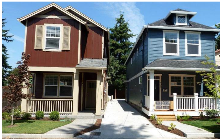
Figure 4-36. Porous pavement that manages only the rainfall it receives can be safely placed adjacent to a building without setbacks. This shared driveway has the added benefit of increasing landscape area. Photo courtesy of Scott Erikson.
