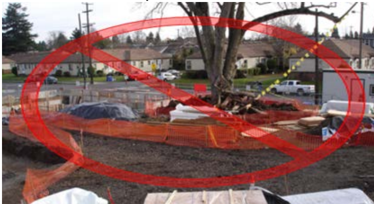
Figure B-9. Orange protection fencing at this project is not deterring stockpiling within the tree canopy. Inadequate tree root protection often leads to health issues that turn a healthy tree into a hazard tree. Tree protection is covered in detail in Chapter 4.
