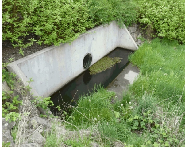
Figure 4-63. This sump settles sediment making it easy to remove and also serves as a headwall to protect pipe integrity. This pretreatment strategy is suitable for high sediment loads but is more difficult to access than other pretreatment strategies presented below.
