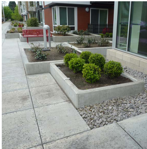
Figure 1-5. Contained planters can be placed on the ground or over impervious surfaces to intercept rainfall and reduce runoff through evaporation.
