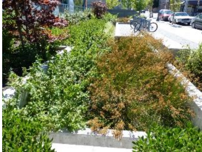
Figure 3-2. A stormwater planter and permeable pavers enhance the RCC/SOU Higher Education Learning Center in Medford, OR. All of the disciplines listed in Table 3-1 might have a stake in this design.
