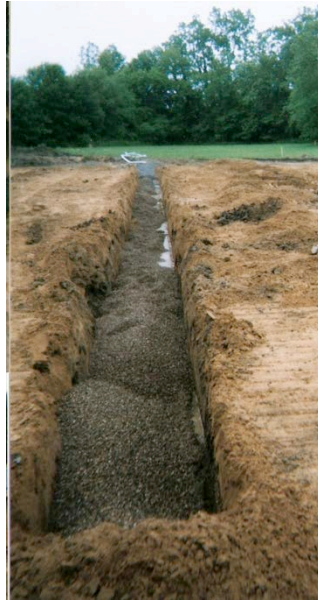
Figure 4-88. Soakage trench during construction. Photo courtesy of Howard's Excavating, New Buffalo, MI.
