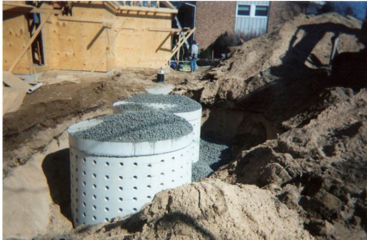
Figure 4-89. Drywells are commonly made of perforated (shown) and sometimes non-perforated (not shown) concrete rings. Photo credit: Howard's Excavating, New Buffalo, MI
