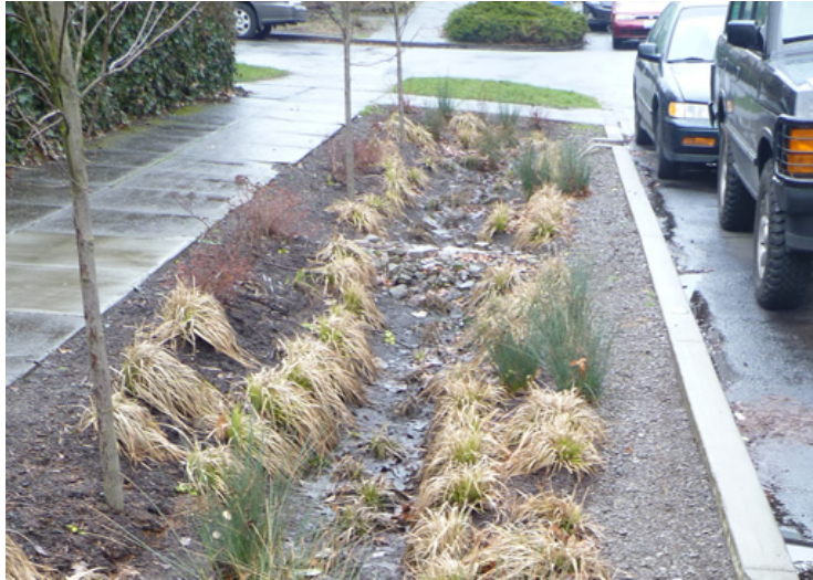
Figure 4-93. Of the three types of swales discussed here, LID swales pond water and provide a higher quality of treatment in a smaller footprint. See Chapter 4 “Rain Garden, Stormwater Planter, and LID Swale BMP”. They tend to be smaller, distributed BMPs compared with other swale types.
