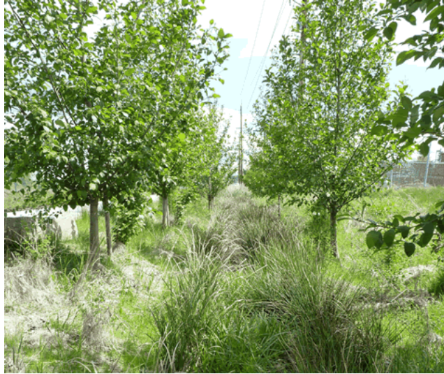
Figure 4-94. Water quality conveyance swales are long, linear facilities that treat stormwater primarily by settling sediments, and the pollutants that attach to them, along their length. Runoff reduction is usually not considered in the design. These facilities are usually less desirable “end of pipe” type solutions, located at the bottom of a project site.
