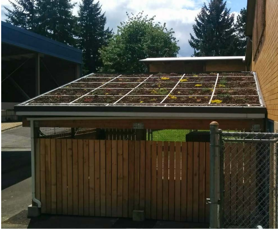
Figure 4-31. Growing medium was stabilized with lumber to keep it from sliding down the steep slope.
