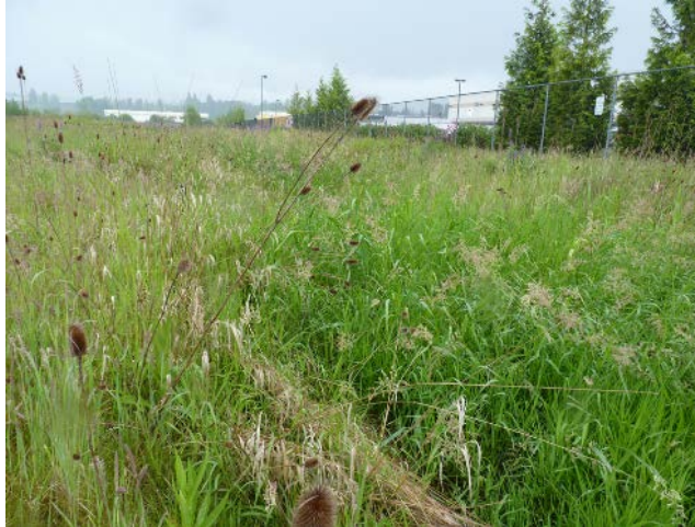
Figure 4-99. Vegetation density down the swale centerline at this industrial warehouse site is ideal. Grasses, shrubs, trees, and groundcover are all suitable for vegetated swales.
