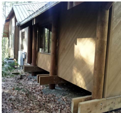
Figure 1-4. Foundations with little to no excavation can reduce runoff from large storms and from areas with high groundwater tables.
