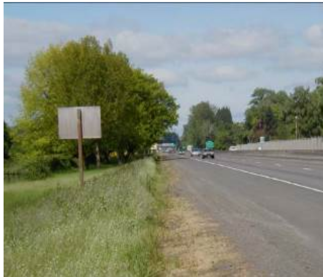
Figure 4-107. Since most highways aren't greater than 75 feet wide from the crown to the road edge, they are well suited for dispersion (aka vegetated filter strips). In this area along a highway in Oregon, excess runoff is likely to flow to a ditch and finally an inlet after leaving the vegetated filter strip. Photo from ODOT Hydraulics Manual 2014, Chapter 14, Figure 6.
