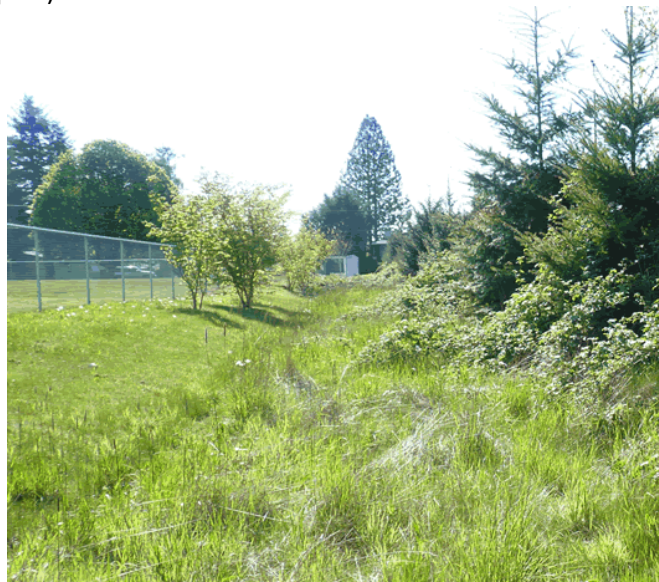
Figure 4-97. This ideal unlined WQ conveyance swale is located away from buildings and other critical infrastructure. Mowing has been performed up to the swale (left); however, the swale itself (unmowed center) is allowed to grow tall and dense. See “Design” below for more information.
