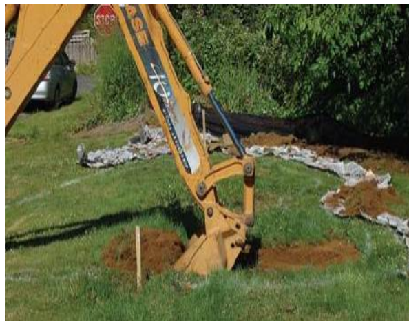
Figure B-10. Avoid foot or vehicular traffic before, during, and after construction. This backhoe is excavating from outside the rain garden, as outlined by the white paint in the grass.
