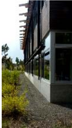
Figure 4-103. There are no gutters on this office building roof. Runoff sheet flows directly over a carefully designed roof edge into a linear rock trench. The exposed concrete at the bottom where water could splash up is a better choice than wood or other materials, that won’t rot and require replacement.
