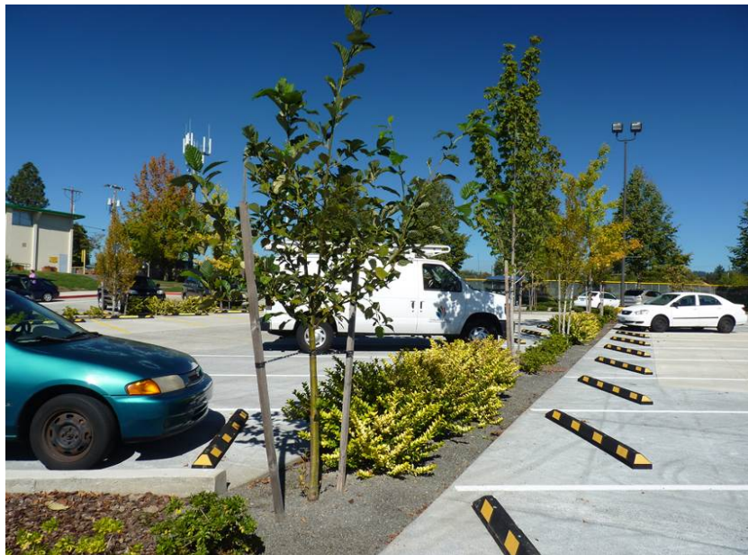
Figure 4-26. This project used structural soil in 4-foot-wide strips underneath the pavement, on either side of the (also 4-foot-wide) planting strip to support traffic loads and healthy root growth. This system (called a Parking Forest www.parkingforest.org ) can be used in existing parking lots to increase canopy without losing parking spaces.
