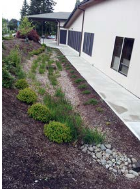
Figure 4-75. This recently installed rain garden retrofit includes a partial liner on the right side and for a distance of about 5 feet out horizontally from the sidewalk. The sidewalk is 5 feet wide, so the 5-foot liner ensures that water cannot infiltrate closer than the recommended 10 feet from the building. The rest of the facility area is able to infiltrate. The vertical portion of this liner runs at least 12 inches deep so that adequate soil volume can be placed on top to grow the chosen grasses. A deeper liner would be needed to plant tall grasses, shrubs, or trees in this zone. The horizontal portion of the liner is installed tipped with 1% slope away from the building/sidewalk, so water can drain out of this area as the rain garden empties. No perforated pipe is needed to ensure proper drainage when the liner is tipped toward a column of soil that can infiltrate.
