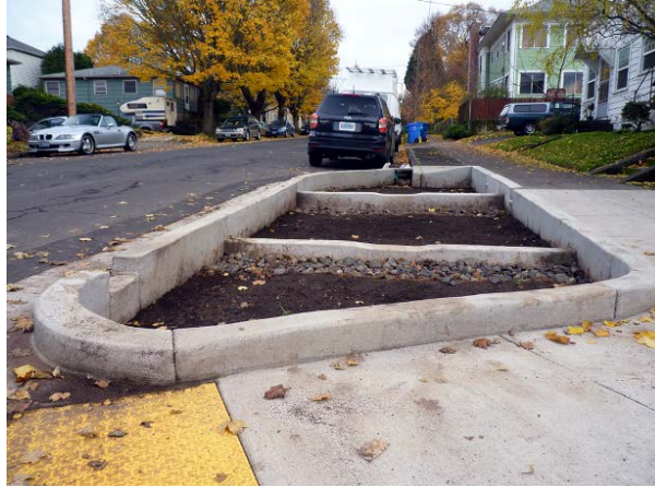
Figure 4-58. An in-ground stormwater planter with concrete check dams in a public street, right before planting. The centerline (looking straight up the center of this photo) slopes at less than 1%. Concrete check dams were needed because the street slopes more than 1%. Grades parallel to the check dam are flat.
