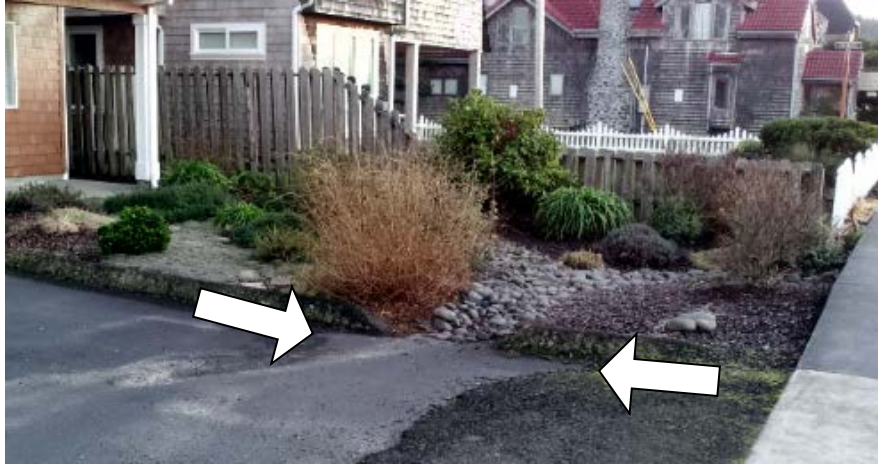
Figure 4-66. Curb cuts are effective where pavement forms a valley gutter that drains toward them. Here, the driveway slopes away from the sidewalk and away from the house making the curb cut the lowest point of the driveway.
