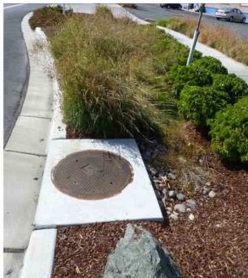
Figure 4-70. This Curb Inlet is ideal to serve as an inlet, pretreatment, and high flow bypass for high sediment areas. A sump in the bottom allows sediment to collect and be easily removed with standard vacuum truck equipment. A slot cut in the back just a bit lower than the gutter line allows water to enter the facility cleaner and with less erosive power than a conventional curb cut. If the bottom of the weir/slot is located at the same elevation as the desired maximum ponding depth, then this will also serve as high flow bypass during large storms, allowing relatively clean water to bypass the facility instead of entering it and causing erosion.
