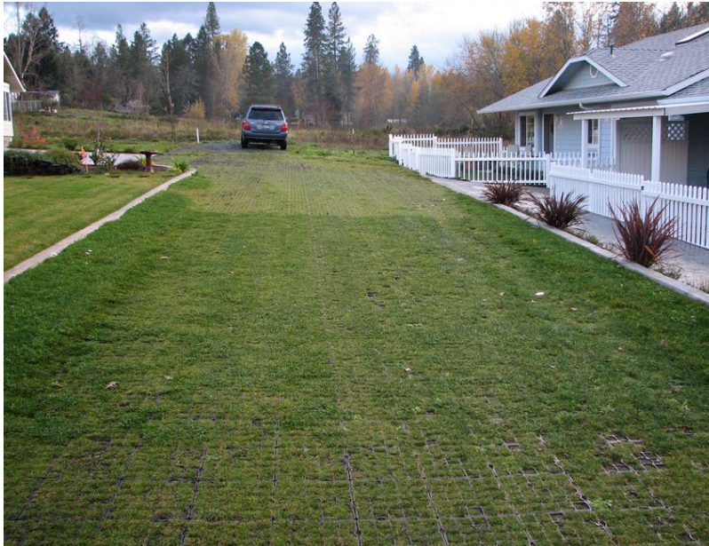
Figure 3-40. Flexible paving systems are often made of plastic grids with numerous openings, as shown here. Photo credit: Teresa Huntsinger
