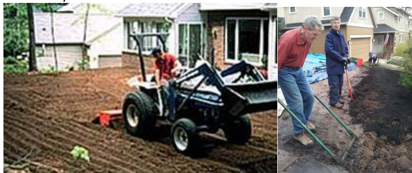
Figure 4-17. A range of construction equipment (cat mounted ripper, tractor-mounted disc, tiller, etc. ) or hand tools such as broadforks and rakes may be used to till and amend soils, depending on the extent of the area to be amended and equipment access.
