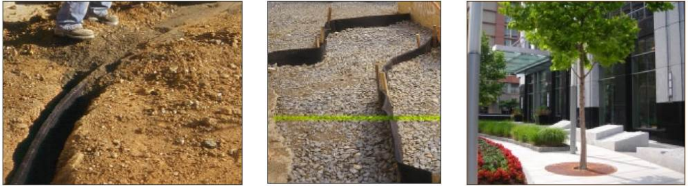
Figure 4-24. Root paths under construction, shown in ground trench (above left) and extending out from a tree space (middle, photos courtesy of James Urban). Root paths run under the pavement to connect tree spaces to landscape areas (above right). Photos courtesy of Casey Trees.
