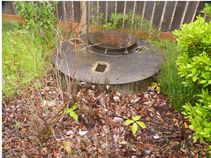
Figure 4-64. When runoff is piped to a facility and there is adequate fall, a sediment manhole can be used in settings with high sediment loads to pretreat runoff before it enters an infiltration vegetated stormwater facility. This facility is a proprietary system that provides advanced treatment for drainage from a gas station’s parking lot and driveways. (The area where gas is pumped is covered and hydraulically isolated and does not drain to this facility.)
