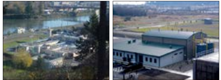
Fishers Lane Water Treatment Plant (left) provided treated water from the Cowlitz River until 2013; the Mint Farm Water Treatment Plant (right) currently supplies treated groundwater
